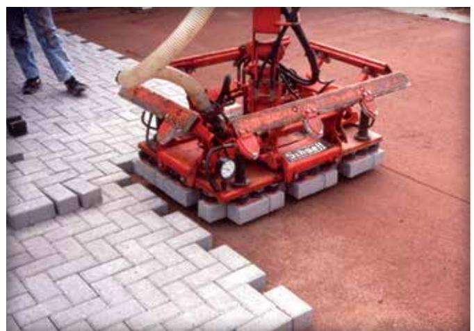
Figure 6. The vacuum head over the paver layer.
