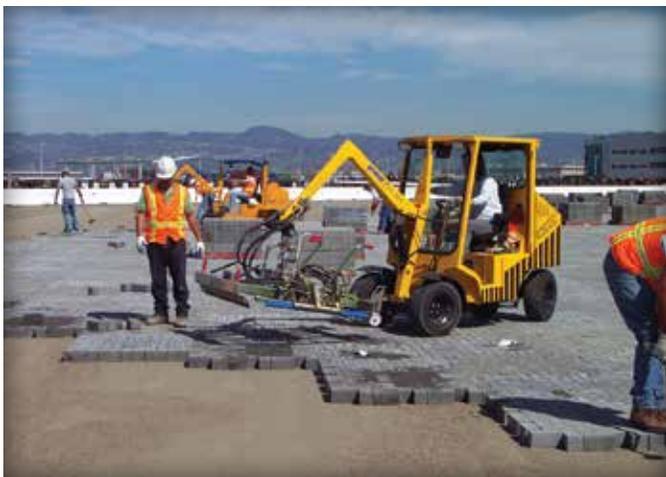
Figure 5. Motorized equipment with a hydraulic clamp.
