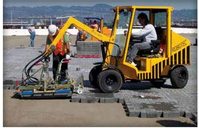
Figure 4. Hydraulic clamp picking up layer of pavers
