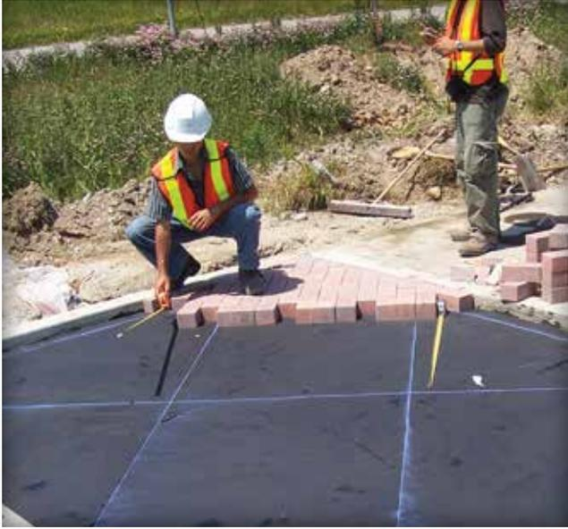
Figure 10. Cut pavers are added along the edges.
