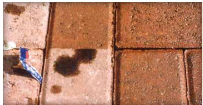
Figure 9. Sealers resist stains which makes them ideal for high use areas where they might occur.
